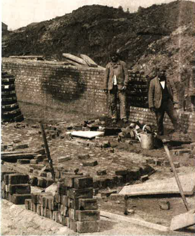
Joseph Bazalgette, standing top right, views the Northern Outfall sewer being built below the Abbey Mills pumping station, c1862
